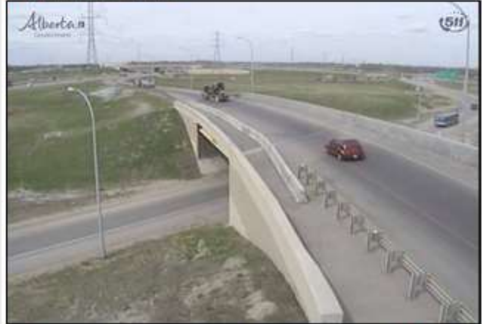
Highway 216 & Whitemud Interchange Near AHD SW-Whitemud
