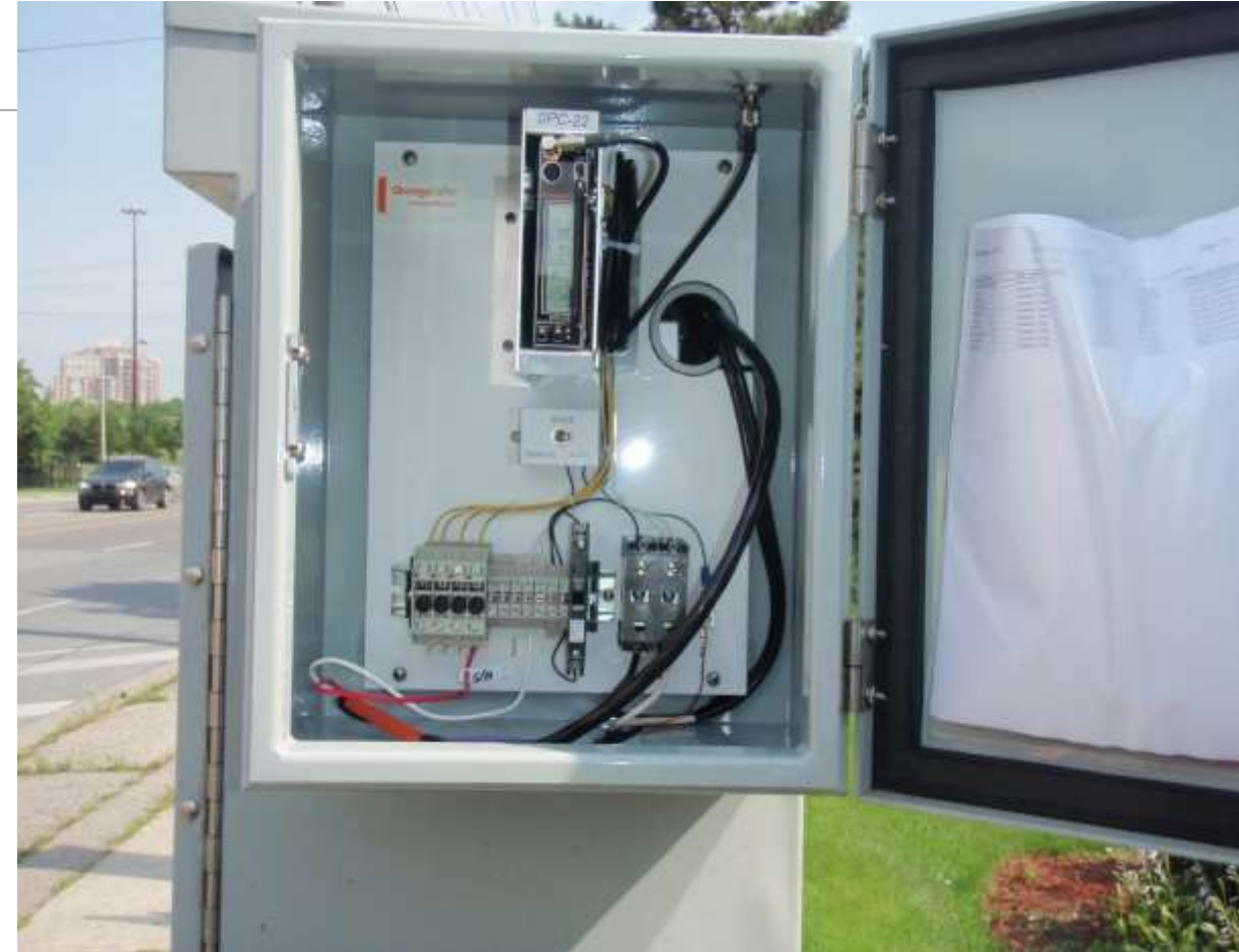
GPS Time Clock Unit Installation
