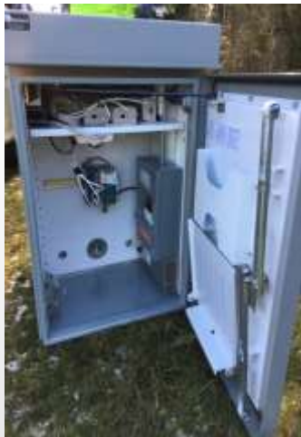
Equipment Install for ITS Testbeds, and Transportation Innovation and Data Labs
