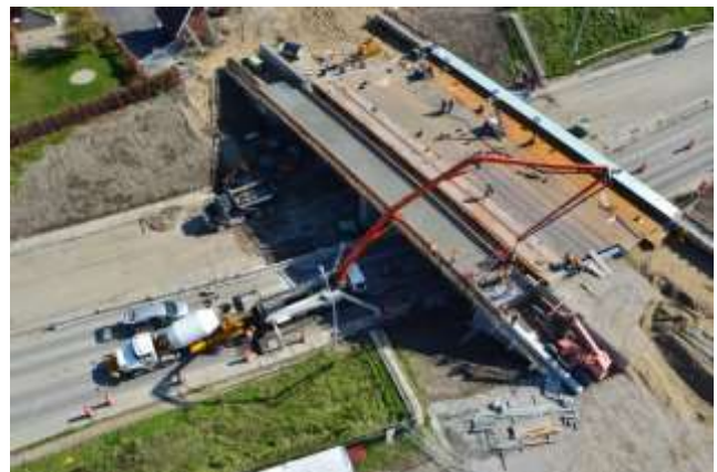
Main St. overpass
